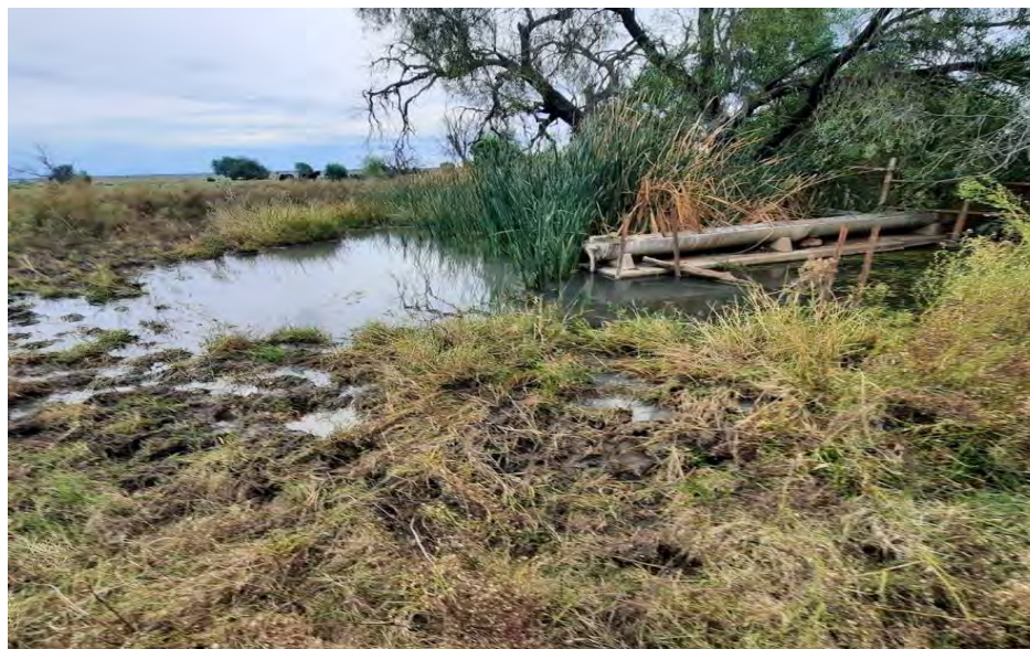
Figure 6: Leaking stock watering trough.
