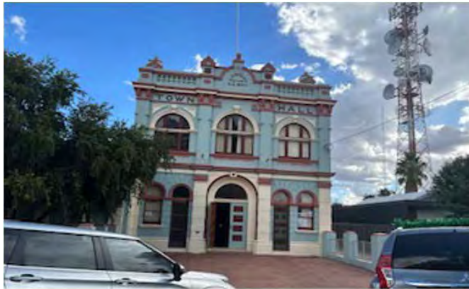
LEFT: Restored Nyngan Town Hall
