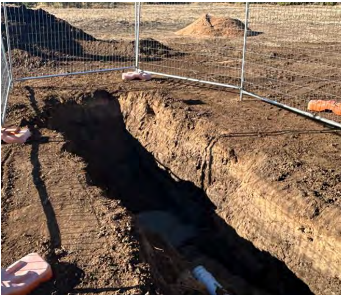
Figure 1: Sewage connection to the core and cluster site (note sewage manhole still to be installed on base slab seen in picture)
