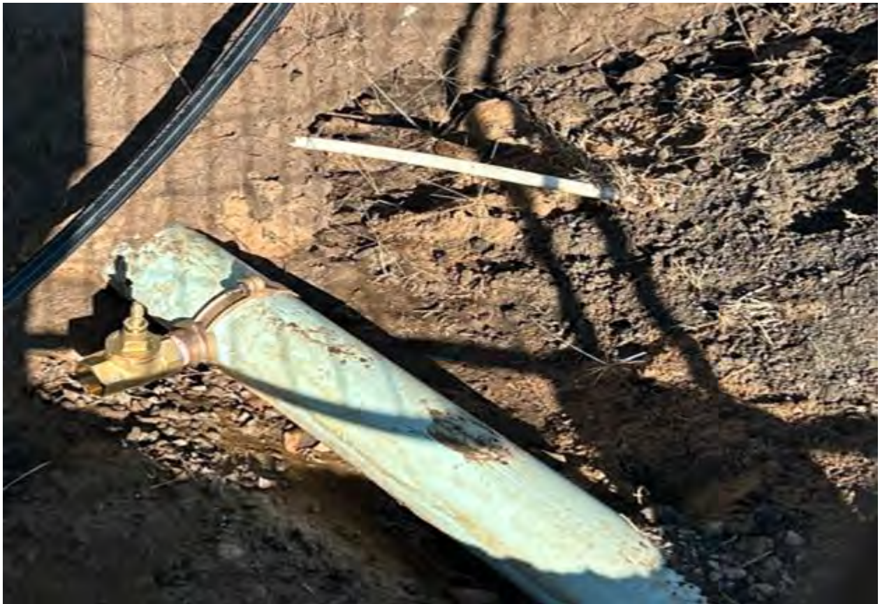
Figure 2: Water connection (40mm) for core and cluster site in Limerick Street
