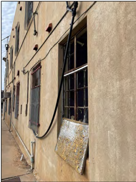
(37) External, central northern window
