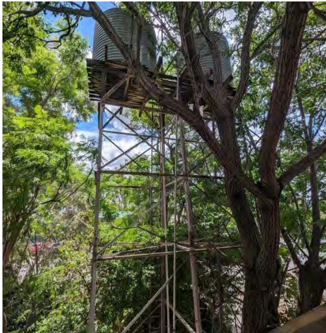
Photograph 35 The water tank viewed from the first-floor fire escape landing on the north wing. The tanks and stands maintain a medium level of significance given their structure and use.
