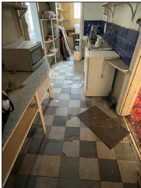
(19) Internal, kitchen cleaning room floor
