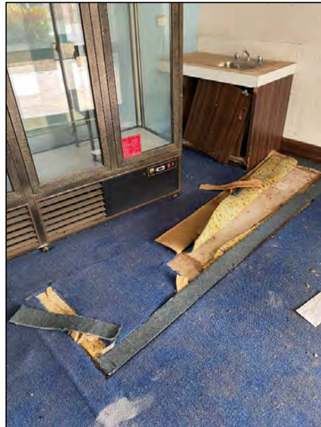
(36) Former travel agent, internal, part floor
