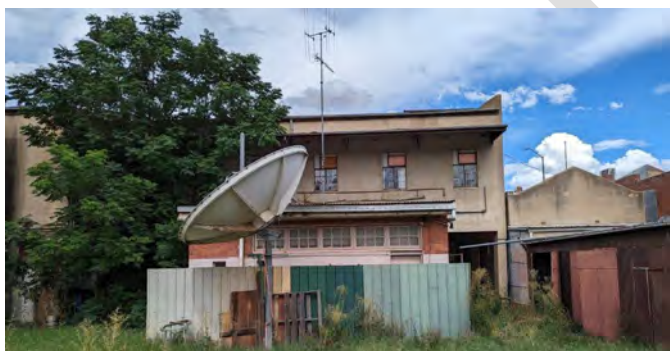
Photograph 46 View of the rear elevation of the Castlereagh wing, noting the later fenced red brick toilet block, which has a low level of heritage significance.
