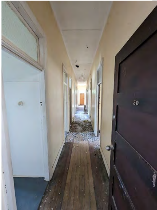
Photograph 143 View within the passage with the bathroom area on the left.
