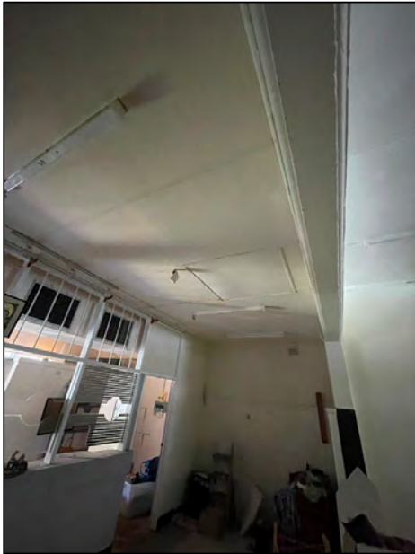
(5) Former hair salon, internal, ceilings and part walls
