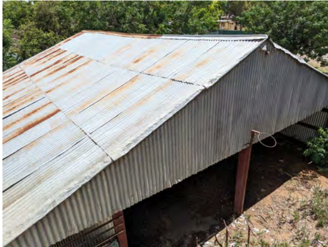
Photograph 39 A view from the fire stair of the central wing of the later shed. The structure has minimal heritage significance.
