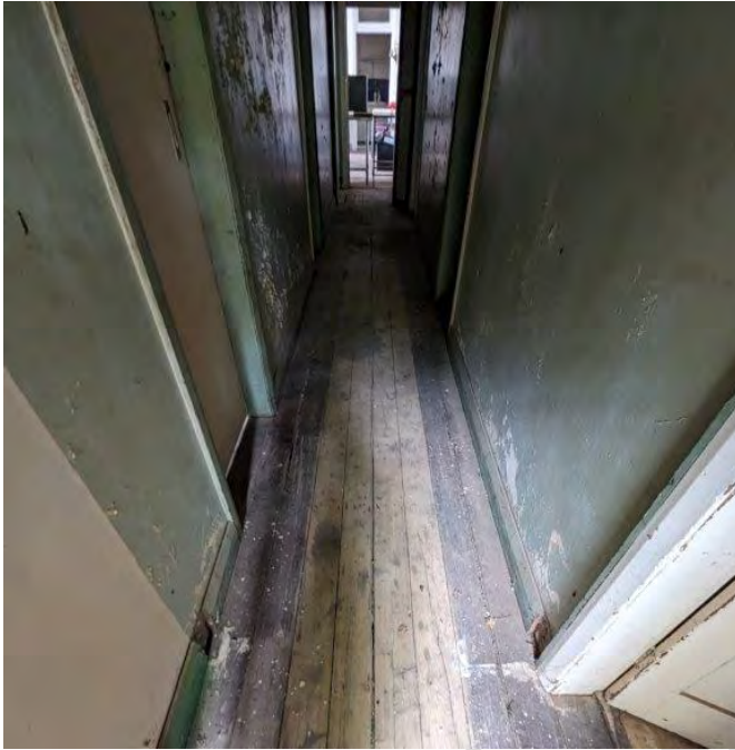
Photograph 84 View from the rear exit back east up the hallway to the kitchen
