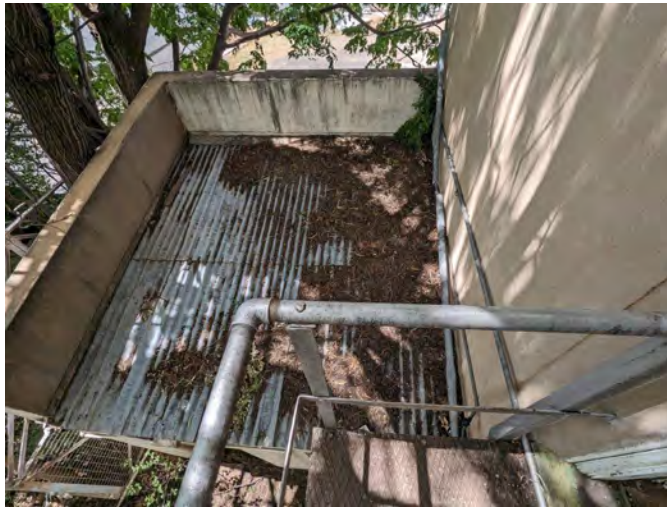
Photograph 121 View from the fire escape landing down to the laundry roof
