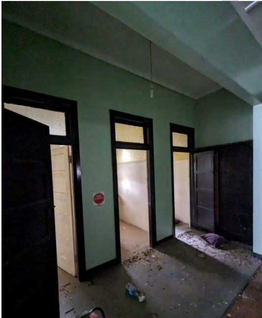
Photograph 137 View of the bathrooms serving the front Castlereagh wing.
