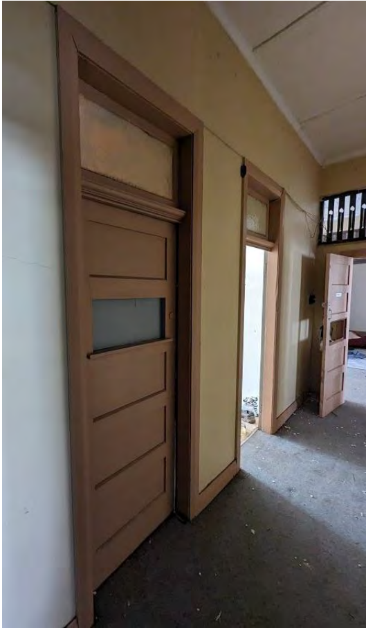
Photograph 123 View looking back north at the entry to this wing and the doors to the kitchen and dining room created from two adjoining rooms on the west side.
