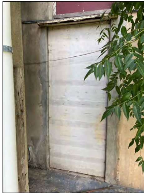
(10) External, men's toilet back door infill panel
