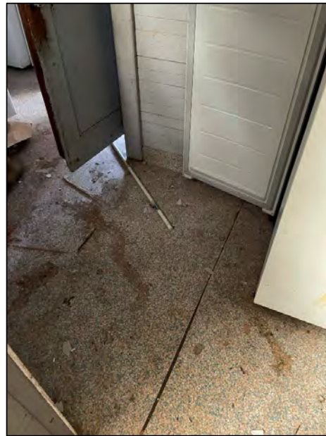
(26) Internal, cool room room floor
