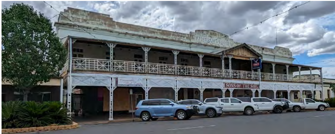
Photograph 8 An oblique view of the front elevation, noting the original cement lettering and date on the façade pediment.
