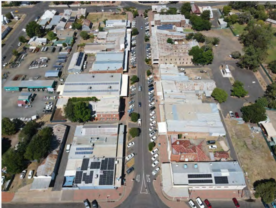
Figure 2: Castlereagh Street, Coonamble, NSW (21.03.2024)
