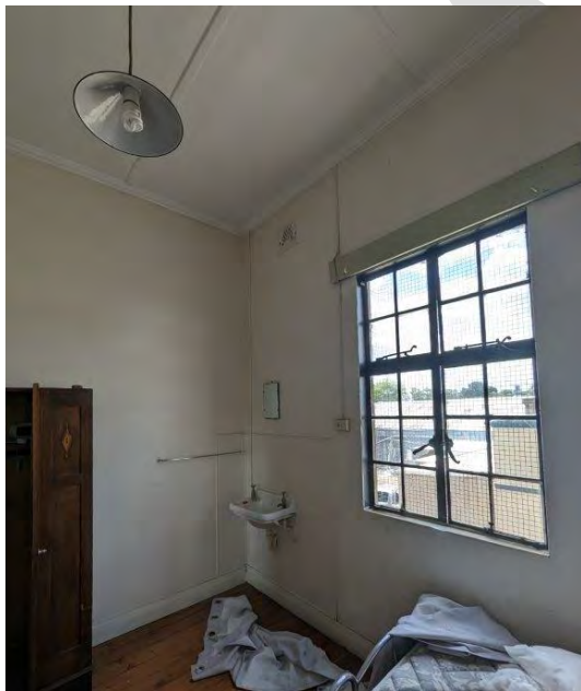
Photograph 114 A view of the north west corner of room 46 to illustrate the hand basin
