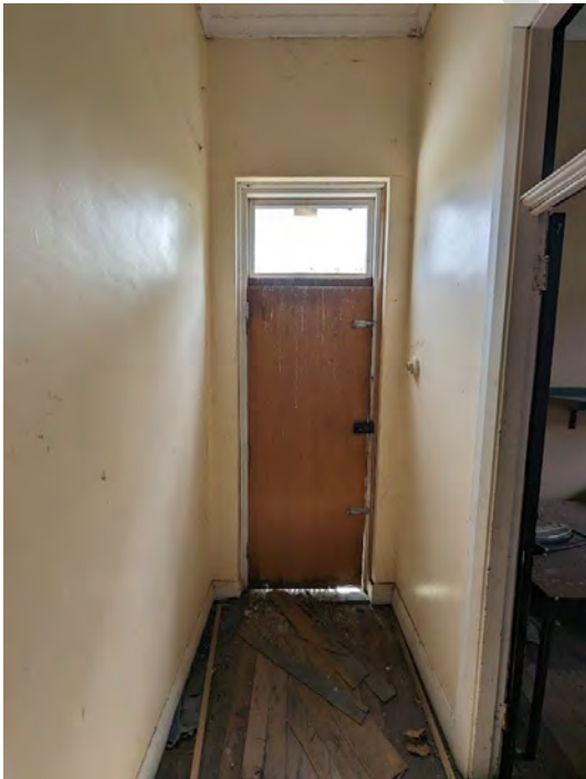
Photograph 149 The fire escape door at the western end of the central extension wing.
