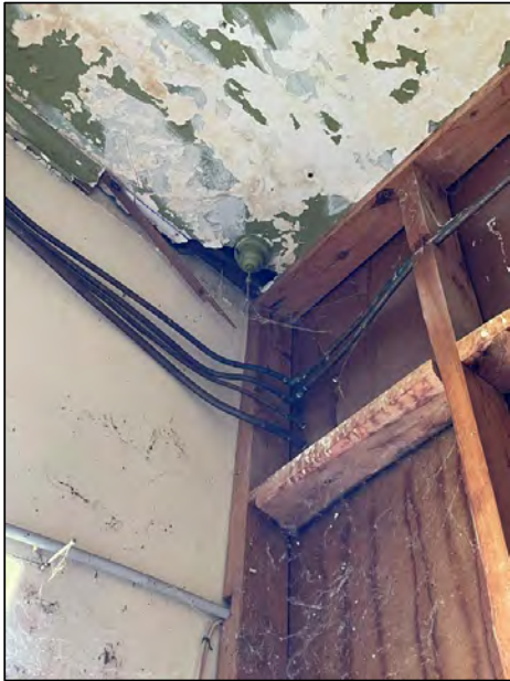
(13) Internal, light fittings throughout
