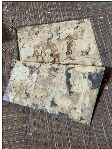
(20) front hallway underlay below carpet squares
