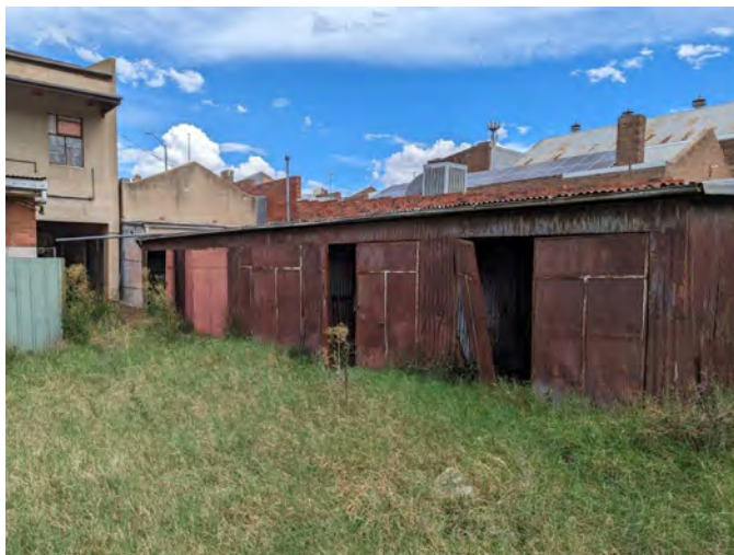
Photograph 45 The steel sheeted garages along the southern boundary, noting the drive through on the left under the main building and where the boundary deviates to accommodate the small shop building. The garages have low level of heritage significance.
