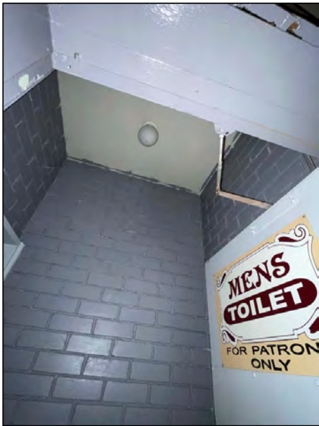
(25) Internal, men's bathroom foyer ceiling
