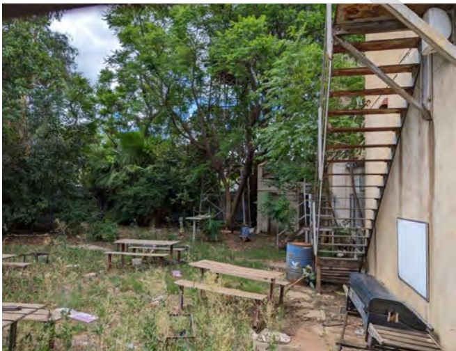
Photograph 34 A view of the yard and West elevation with fire staircase and laundry from the north wing beyond. The overgrown tree requires removal to reduce the impact of the roots on the building.
