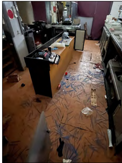
(22) Internal, main bar floor
