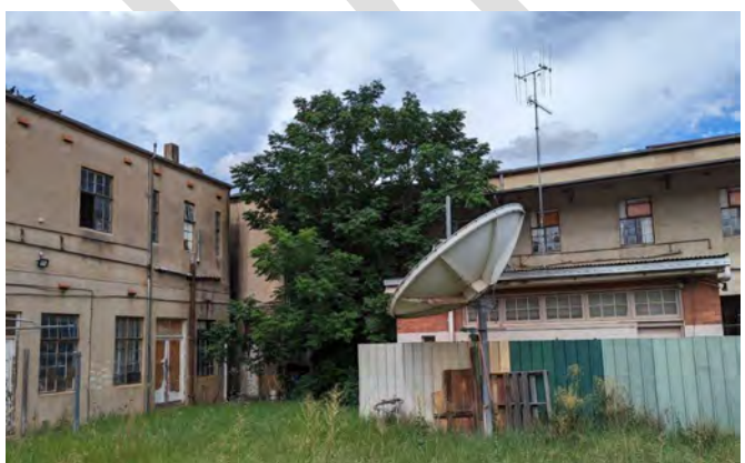
Photograph 47 View towards the north east showing the south elevation of the later central extended wing. The wing has a lower level of heritage significance and is not in the same condition as the other two wings due to pigeon infestation on first floor and water damage to the ground level. The overgrown tree requires removal to reduce the impact of the roots on the building.
