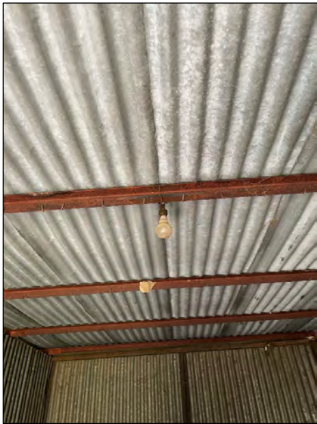
(1) Carport, internal, light fittings
