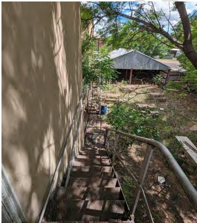
Photograph 36 View to the south from the first-floor fire escape of the rear yard including the end of the central wing with its fire stair and the shed which adjoins the stable. The shed is an later structure with minimal heritage significance.
