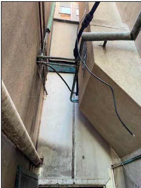
(11) External, rear entrance adjacent boiler room, wall
