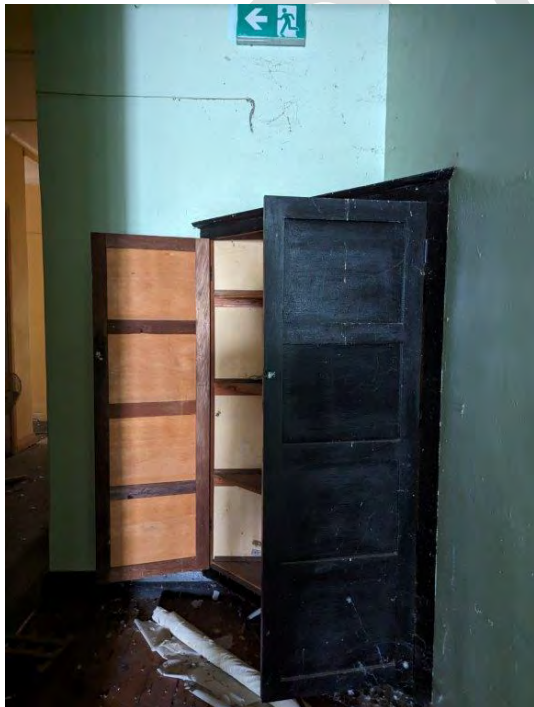
Photograph 127 Built in joinery located at the change in room widths.
