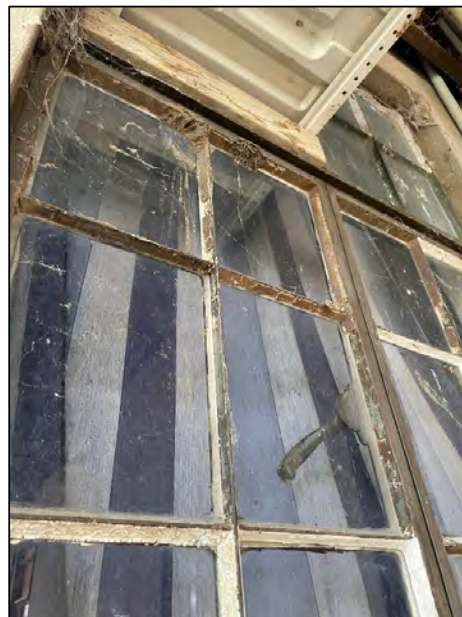
(40) External, 1 st floor southern window
