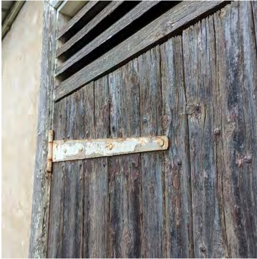
Photograph 30 Hardware and joinery construction with upper louvre vent.
