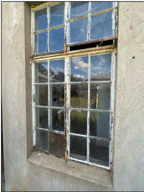
(9) External, window putty. Further investigation is required
