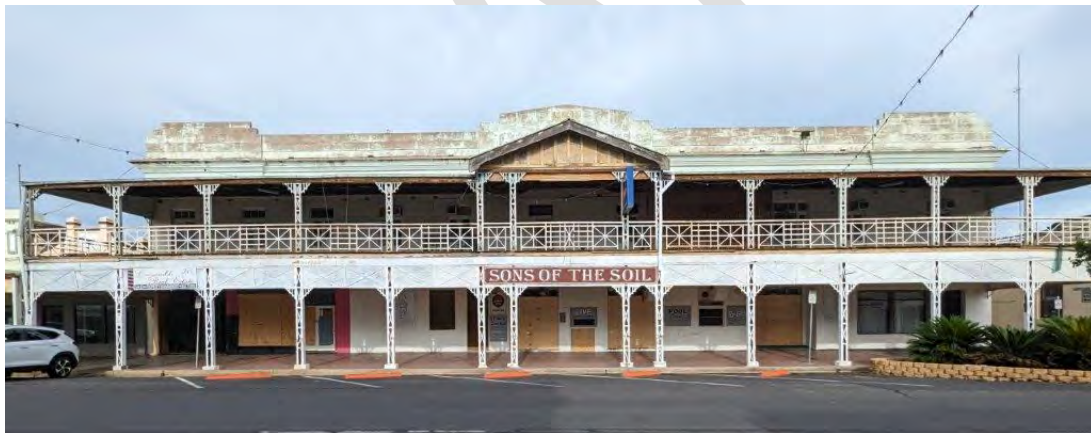
Photograph 7 The full East elevation to Castlereagh Street, noting the original verandah, drive through at the last southern bay and the rendered facade.
