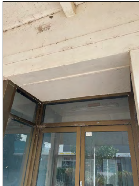
(34) Former travel agent, external and internal, foyer ceiling
