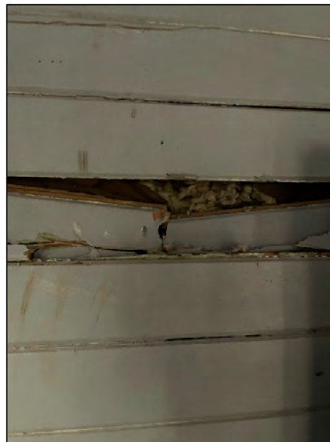
(28) Internal, cool room wall insulation
