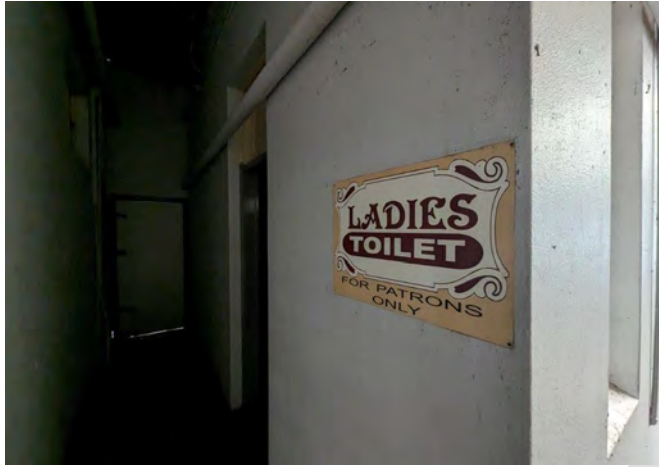
Photograph 89 The eastern end of the ground floor extension was adapted to provide female toilets.
