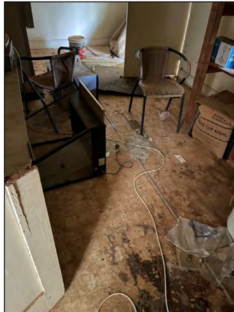
(16) Internal, rear storage room floor
