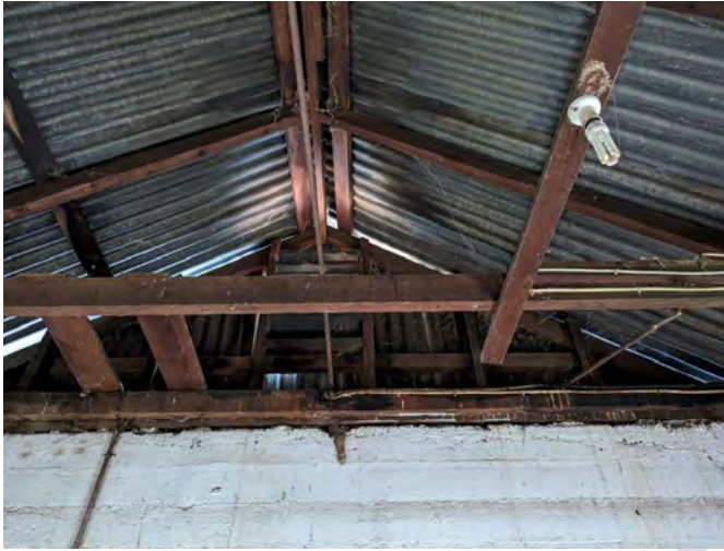
Photograph 28 View of the gable end to the roof with louvre vent.
