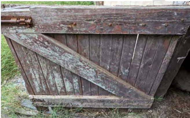
Photograph 31 Hardware and lower door construction.
