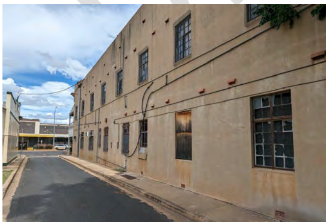
Photograph 50 A long view of the North elevation, noting the general conditions, steel framed windows and services.
