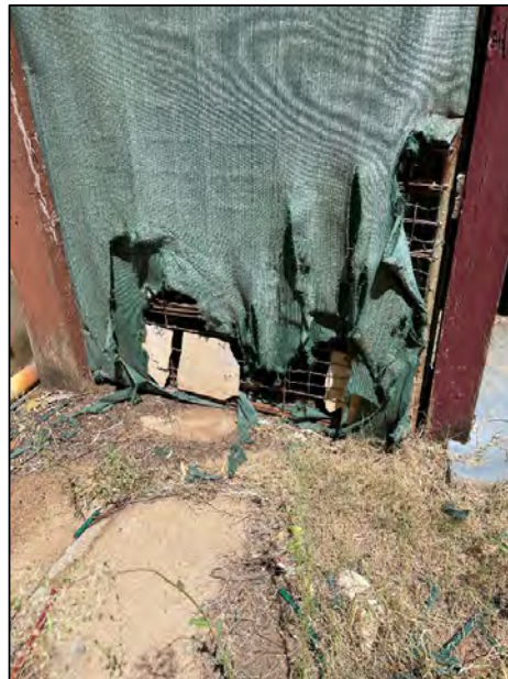
(8) External, rear gateway, infill panels
