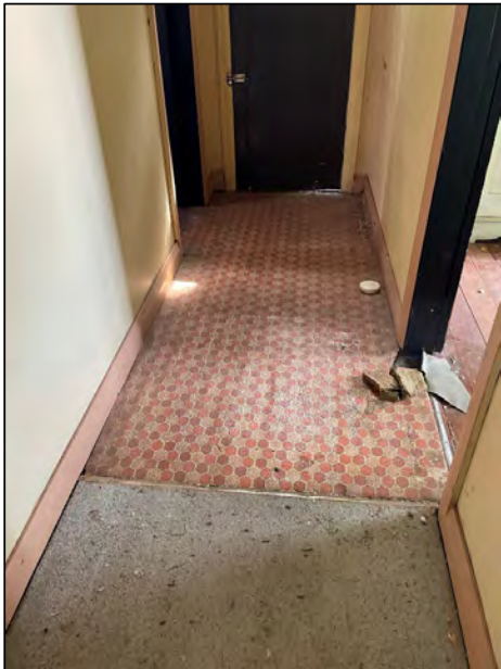
(31) Internal, 1 st floor northwest entrance floor
