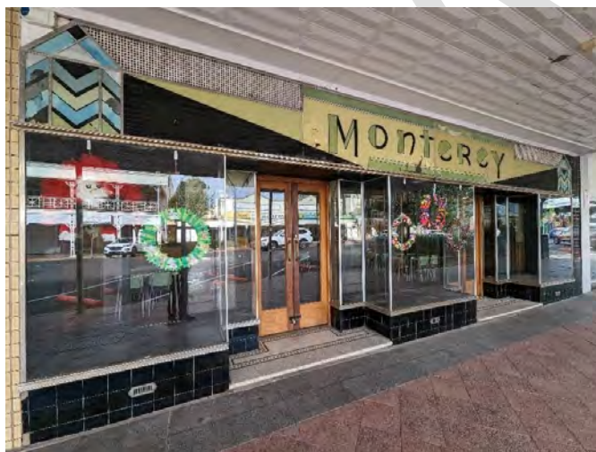
Figure 4 External shopfront to Monterey Café, noting restored materials and details from 2023
