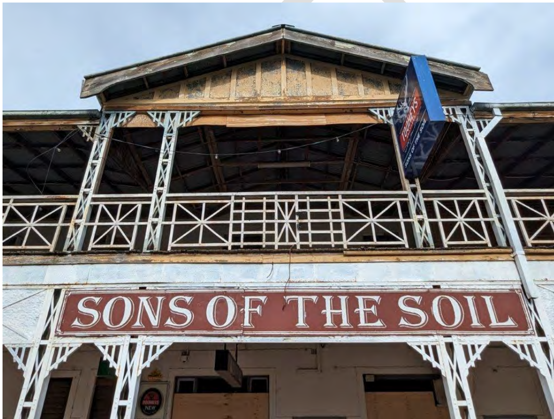
Photograph 9 The gabled pediment in the verandah façade provides the symmetrical feature on the elevation. The early Butlin Archive images indicate that the structural details to the verandah are original.
