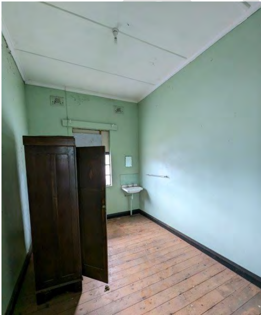
Photograph 133 The end room on the west side of the main wing.
