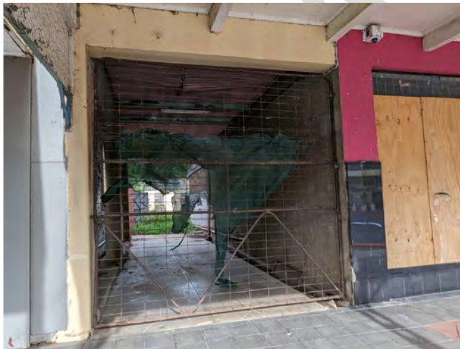
Photograph 12 View of the drive through which gives access to the southern yard with the stable, open steel garage to the southern boundary and steel shed to the western boundary.
