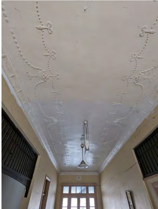
Photograph 103 Detail of the decorative plaster ceiling. Note the original light fitting.
