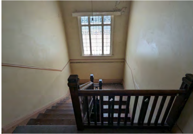
Photograph 100 A view from the upper landing, noting the decorative leadlight window. Note the minor water damage in the top corner of the wall.
