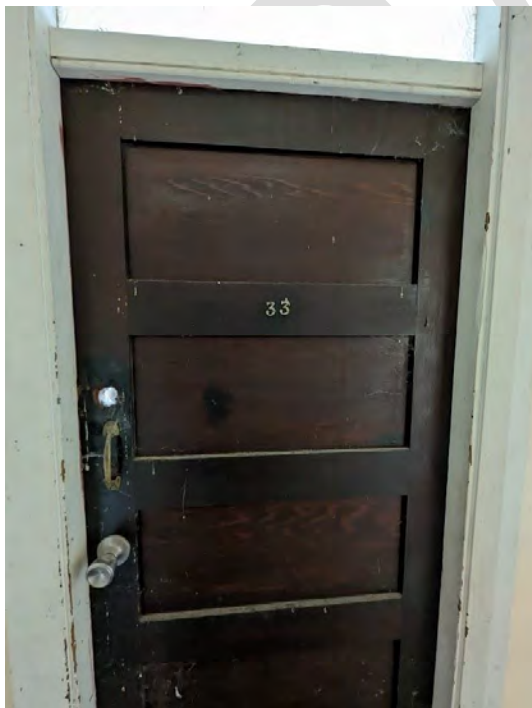
Photograph 145 Typical guest room entry door in this wing.
