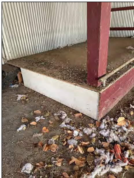
(3) Covered dancefloor, infill panel
