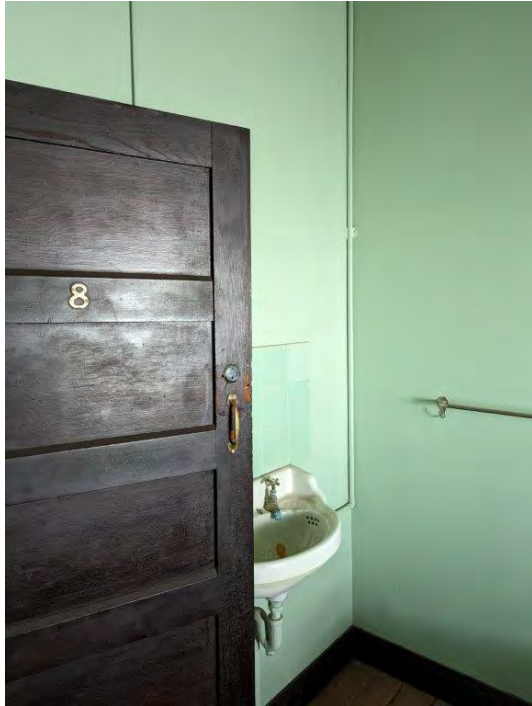
Photograph 130 The original handbasin.
