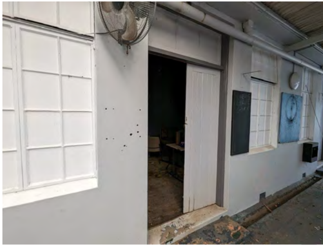
Photograph 92 The central room of the north side of the extension wing
