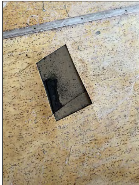
(32) Internal, 1 st floor staff kitchen floor vinyl and underlay
