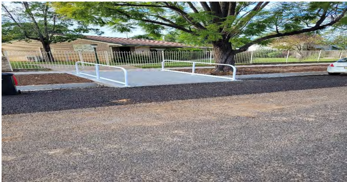
Figure 2 Completed civil works at the Towri Units
