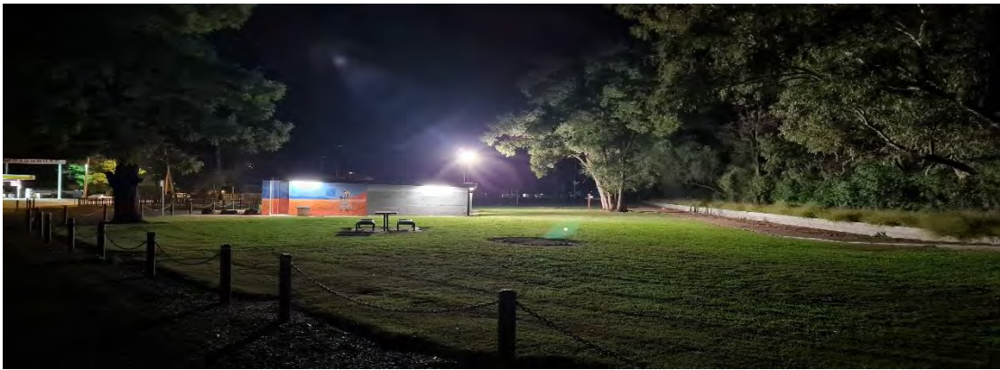
Figure 1 Upgrades to lighting in Smith Park, Coonamble.
