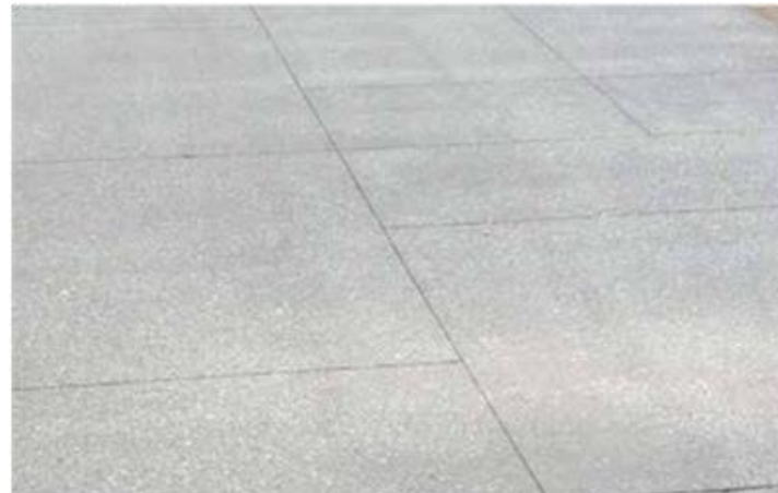
Concrete pavement with light honed finishes - $140 mln + gst supply and Install) to pedestrian areas / $175 mln to vehicular cross overs
