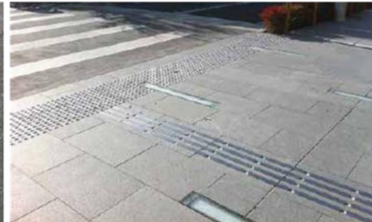
Granite pavers (600x300x40) - $110 mln + gst. (supply only) $415 m2 supply / Install with conc base
