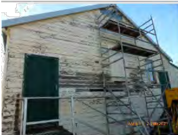
Repaint/Re-clad Hall Exterior Walls - Quambone
