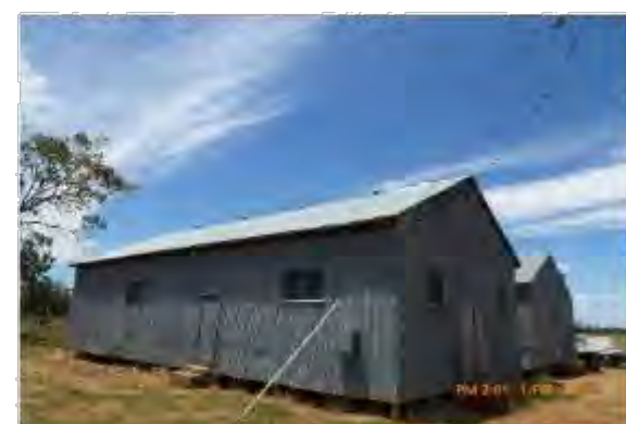
Install/replace Grab Rails/ Hand Rails and entrances.
