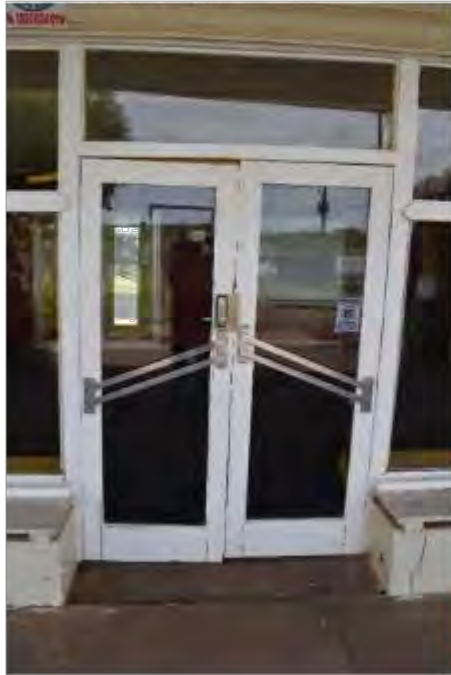
Clean Up Interior/Replace doors
