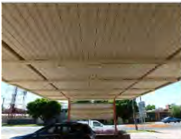
Under Cover Parking
