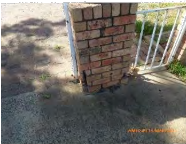
Front fence brick work repairs
