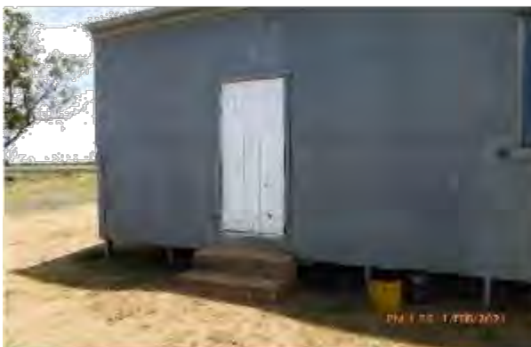
Replace doors and window gauze
