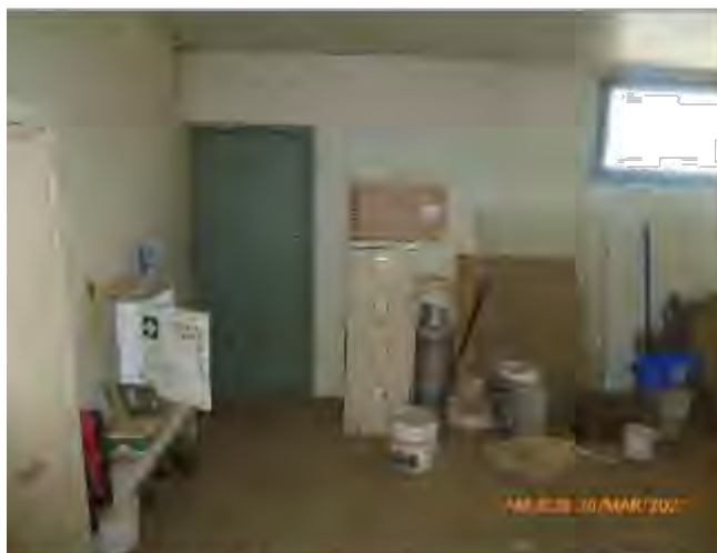
Clean up and paint job
