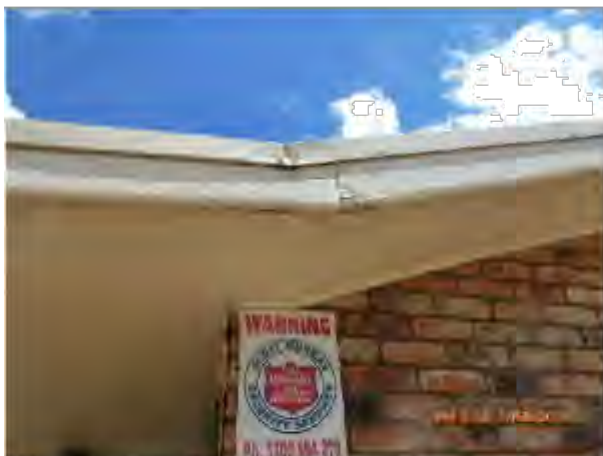
Minor Repairs to Eaves and side boards
