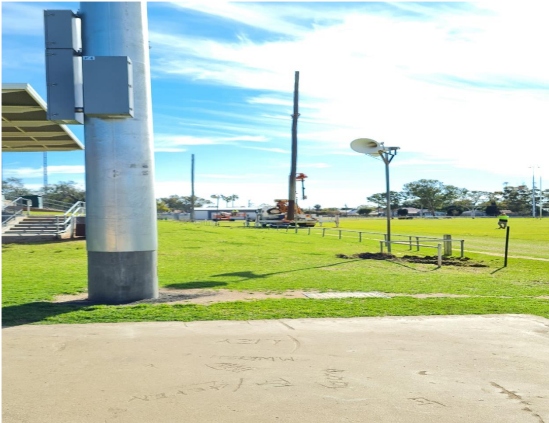
Removal of old lighting tower at the Coonamble Sportsground
