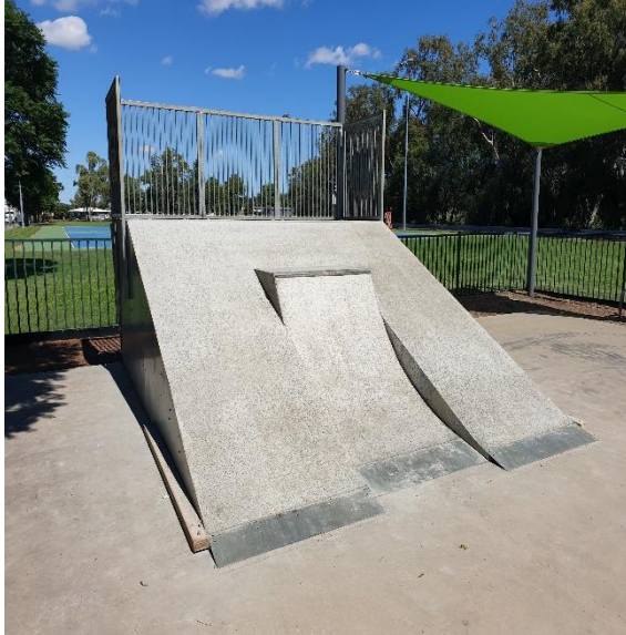
Repaired Skate Module
