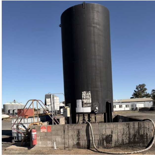
Figure 5 - Existing Bitumen Tank
