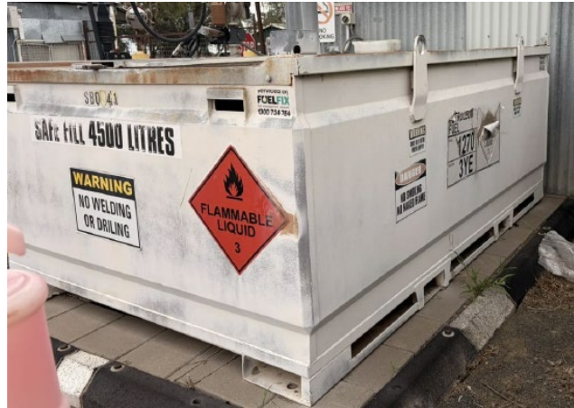
Figure 4 - Existing ULP Tank
