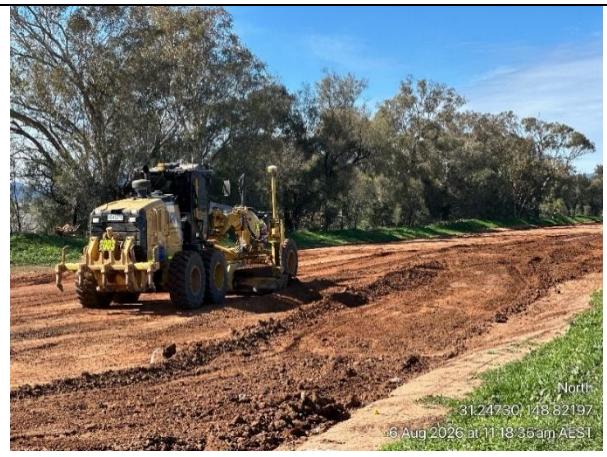
Placement of Earthworks Layer 1 Segment 1
