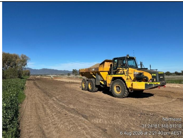
Placement of Earthworks Layer 1 Segment 1
