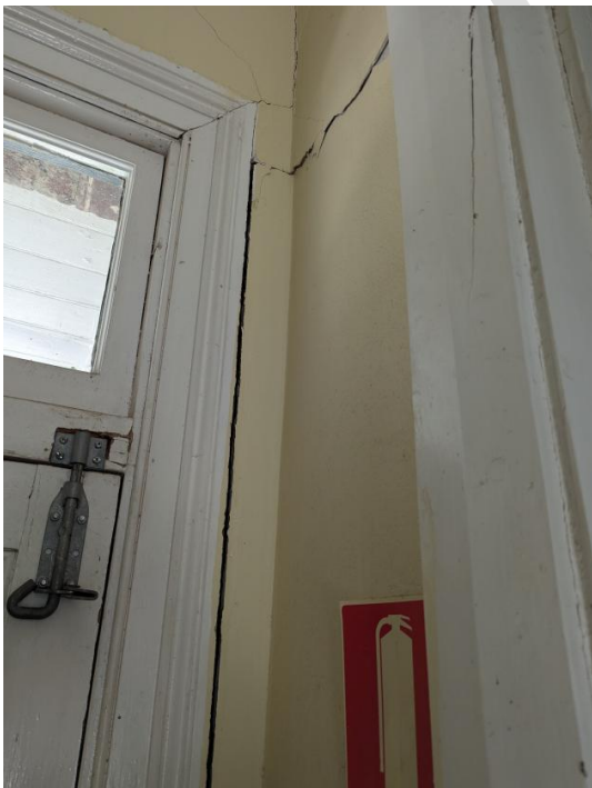
Photo 24 Following remediation, cover moulds to be used to conceal backing rod insertion and sealant next to door
