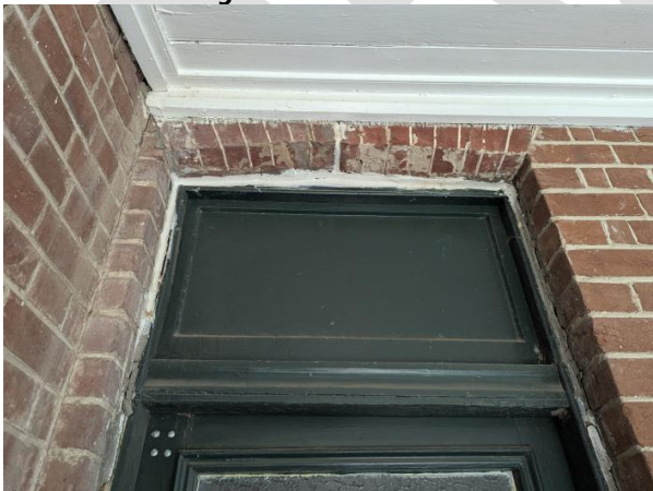
Photo 13 As above noting sealant strategy
