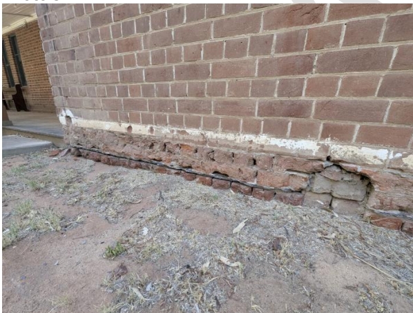
Photo 6 Brick replacement with suitable recycled bricks
